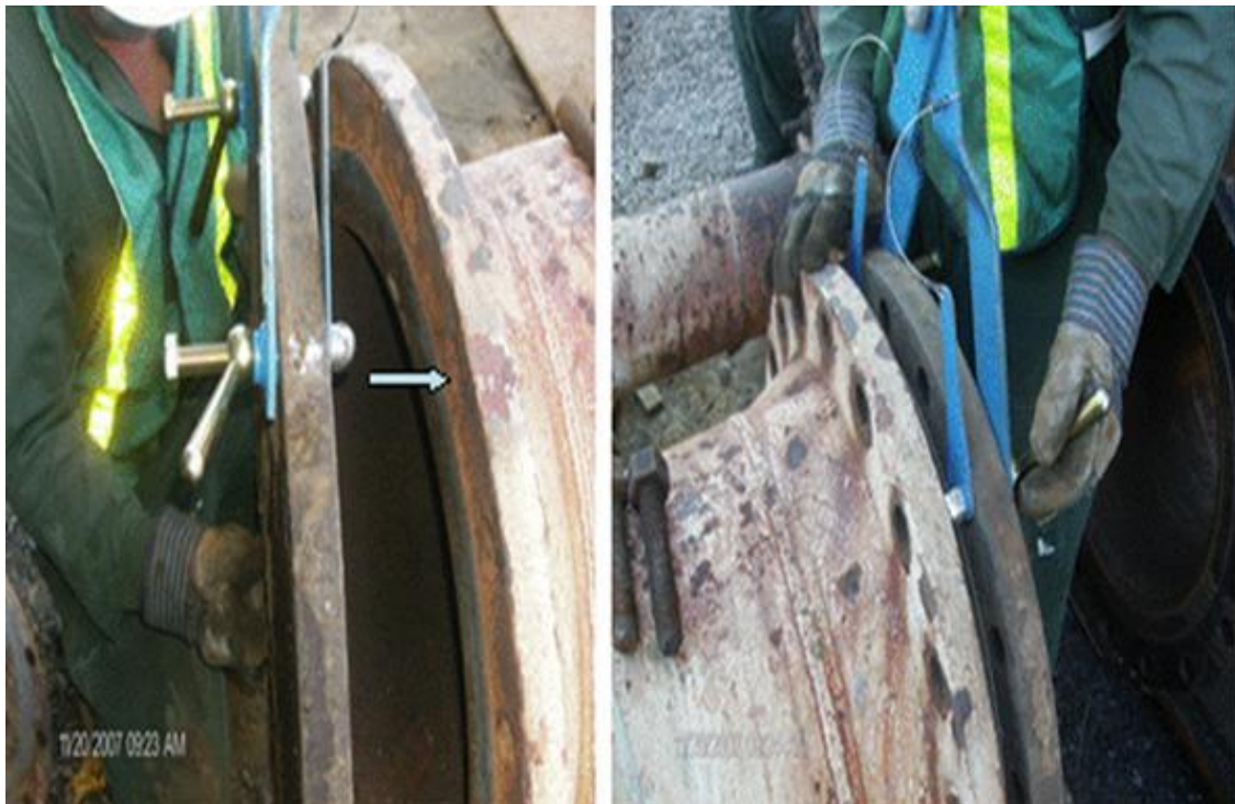
Guide Line-up Lugs into Flange Hole
