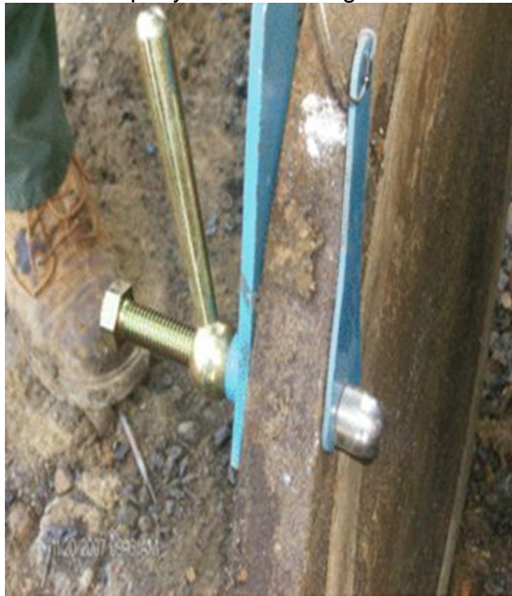
Properly Installed Flange Jack
